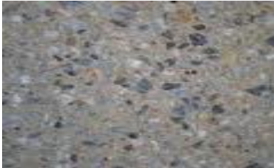
Figure 1: Sand blasted concrete
