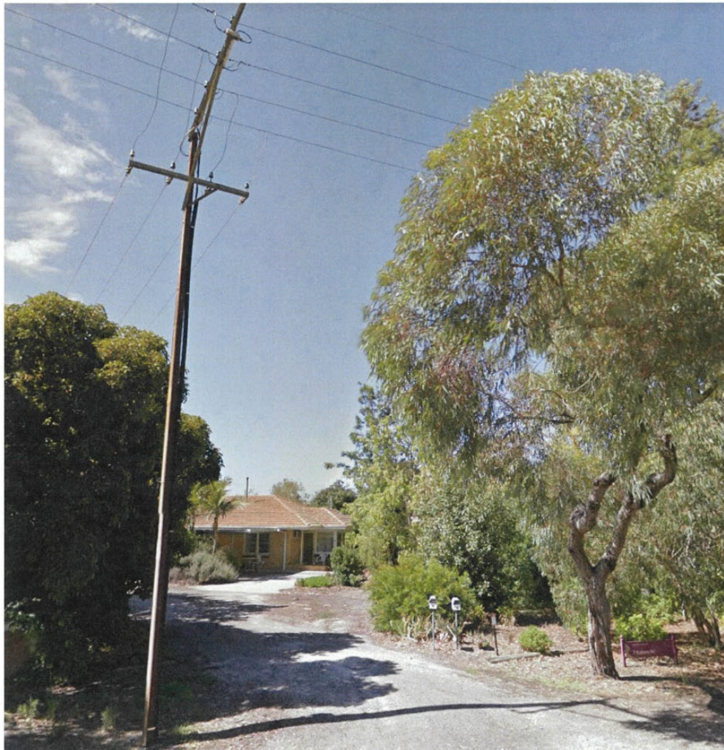
Existing power line adjacent current access.
