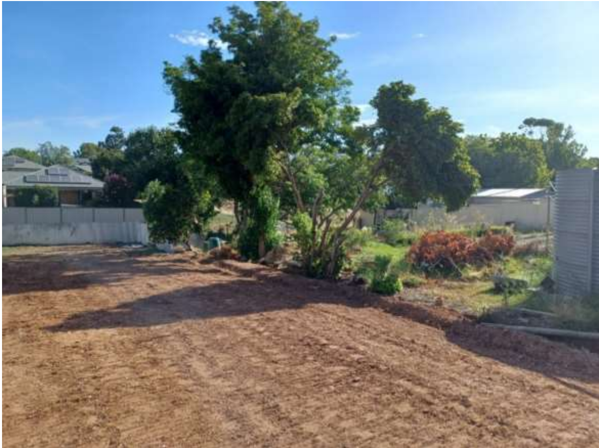
Figure 9: Site Photo – looking south-west from subject site
