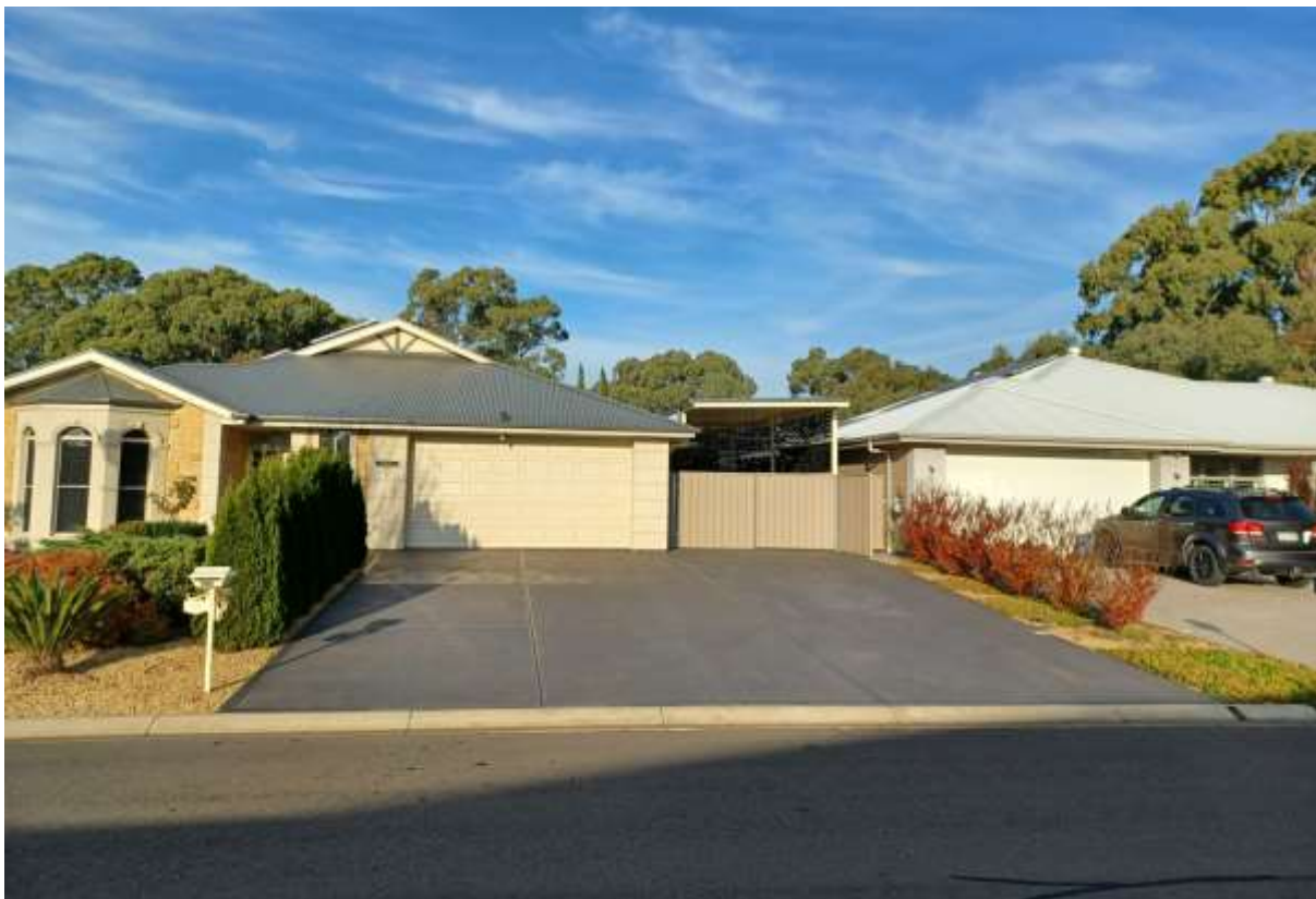
Figure 4: Looking east from Fairbrother Circuit
