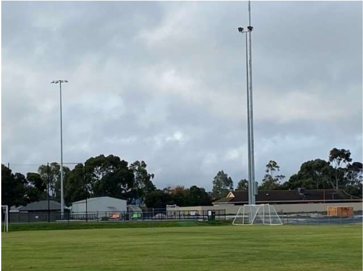
Figure 7: Looking north within the site toward pad for the new clubroom
