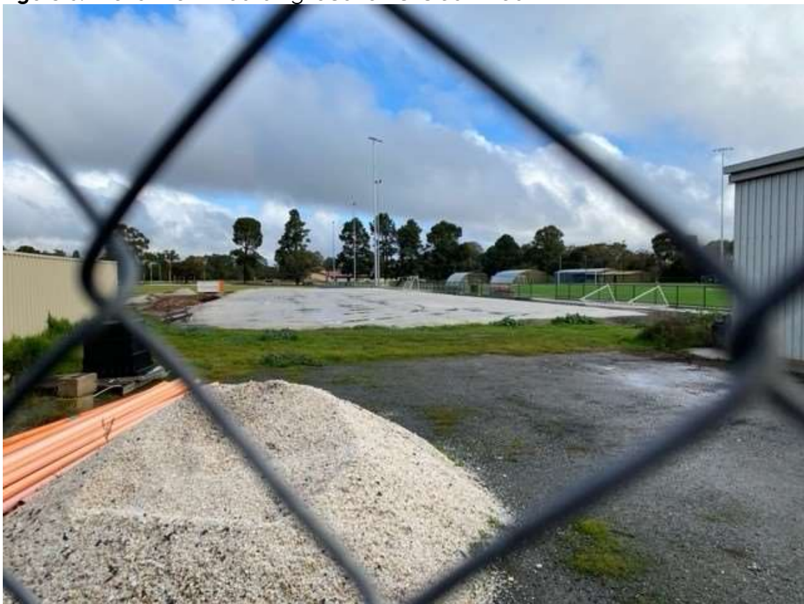
Figure 6: Looking south toward pad for the new clubroom
