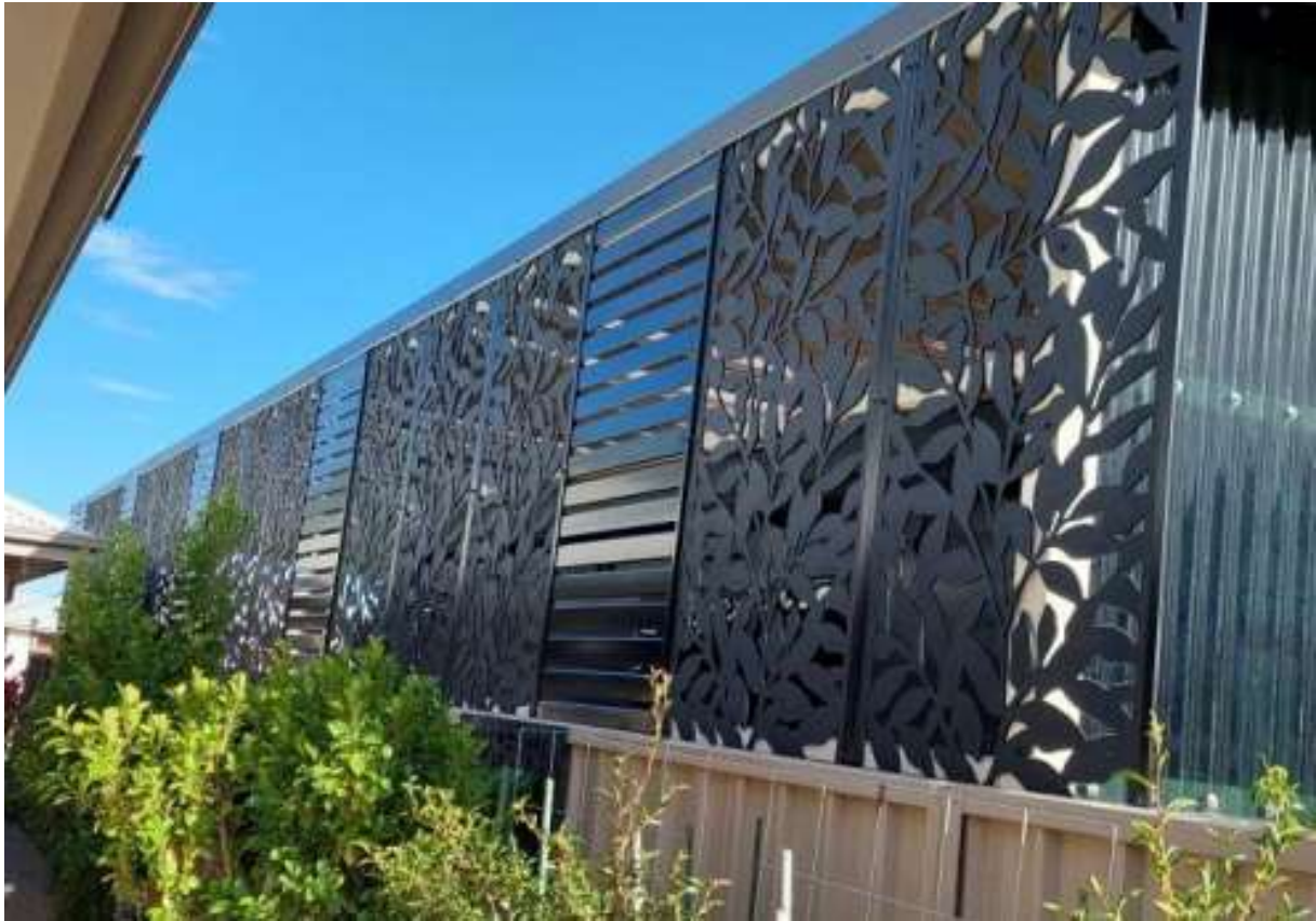
Figure 5. Looking north-east from side yard of 19 Fairbrother Circuit
