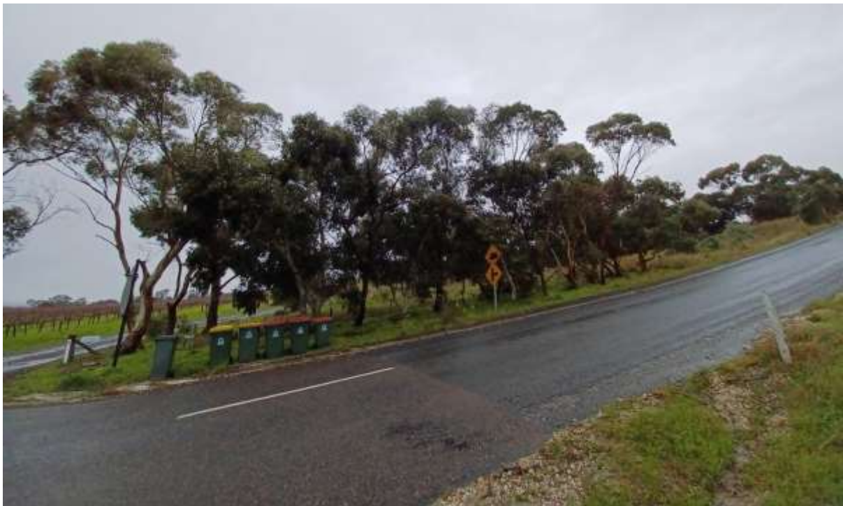
Figure 4: Site Photo – standing opposite site driveway on Rifle Range Road, looking north-north-east at subject site
