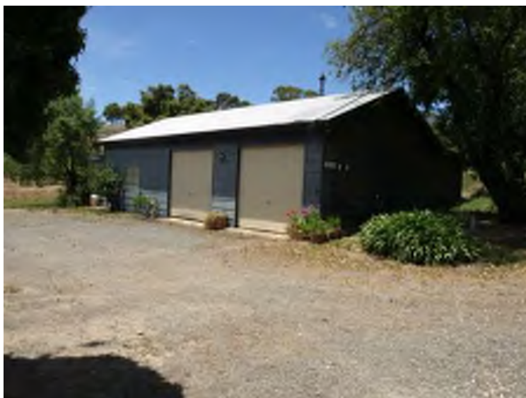
Photo 18 Existing Garage – overhanging branches are to be removed.
