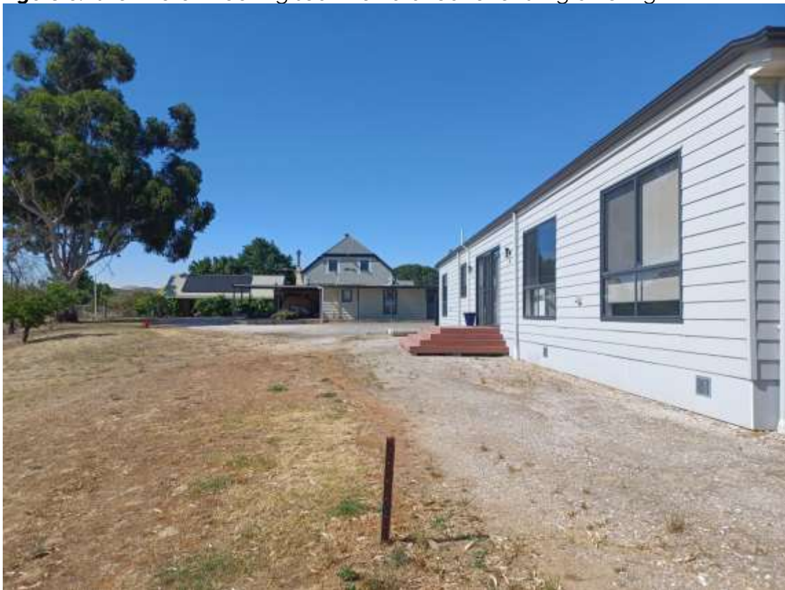
Figure 9: Site Photo – Looking north toward rear of existing dwelling
