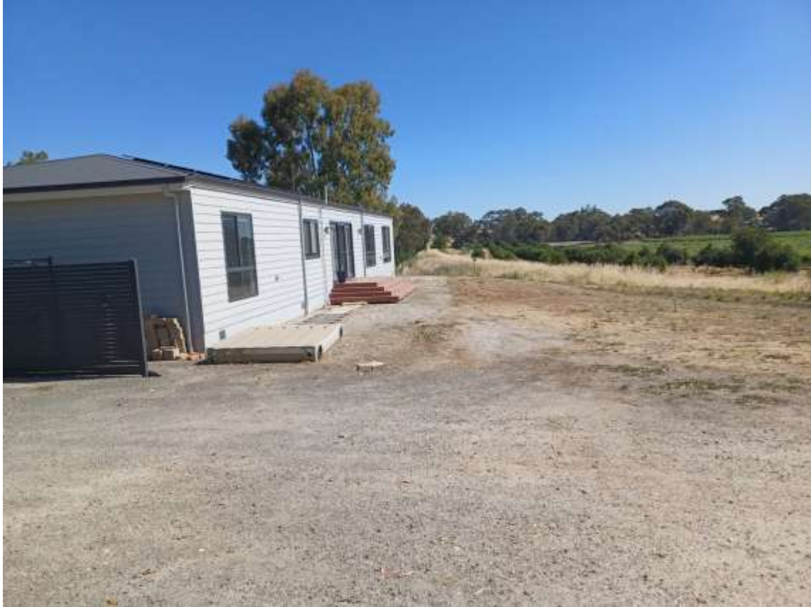
Figure 8: Site Photo – Looking south toward rear of existing dwelling
