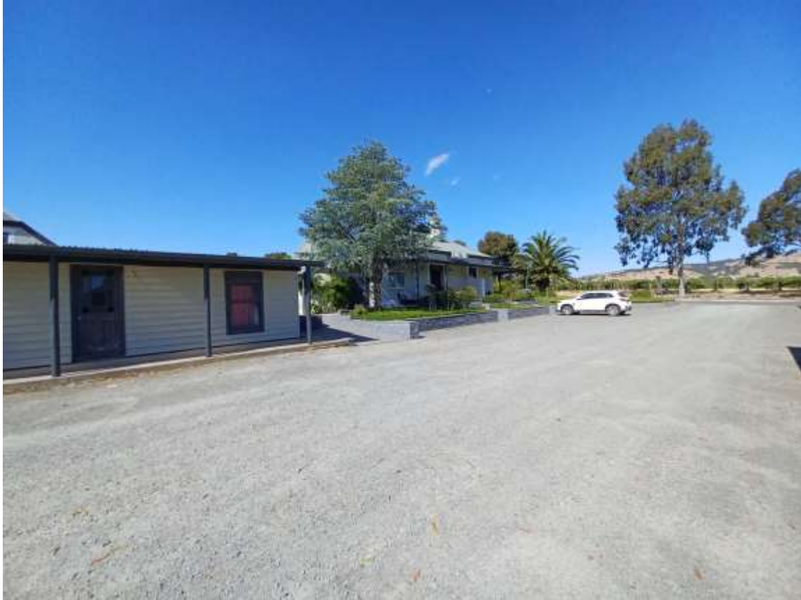
Figure 10: Site Photo - Existing accommodation and laundry/store
