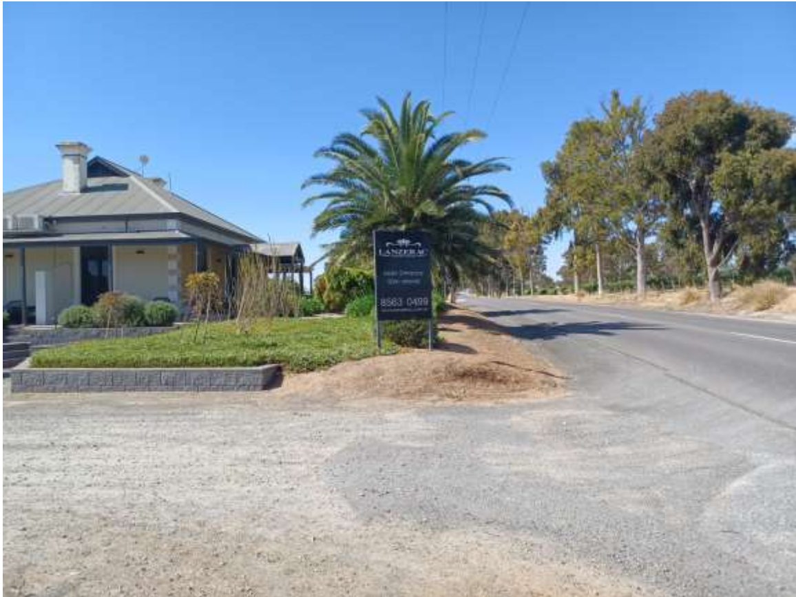
Figure 16: Site Photo – Menge Road frontage, view north
