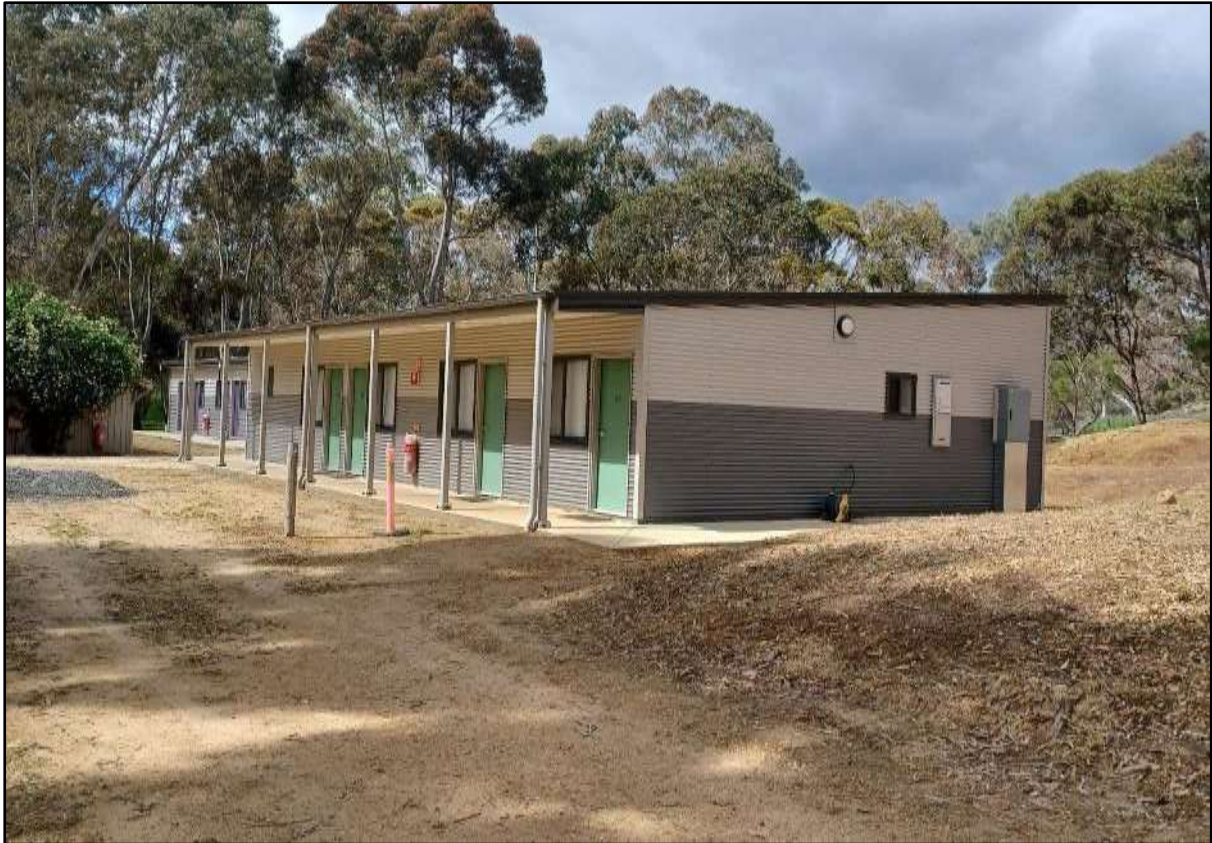
Figure 7: Site Photo – Dormitory D, already replaced
