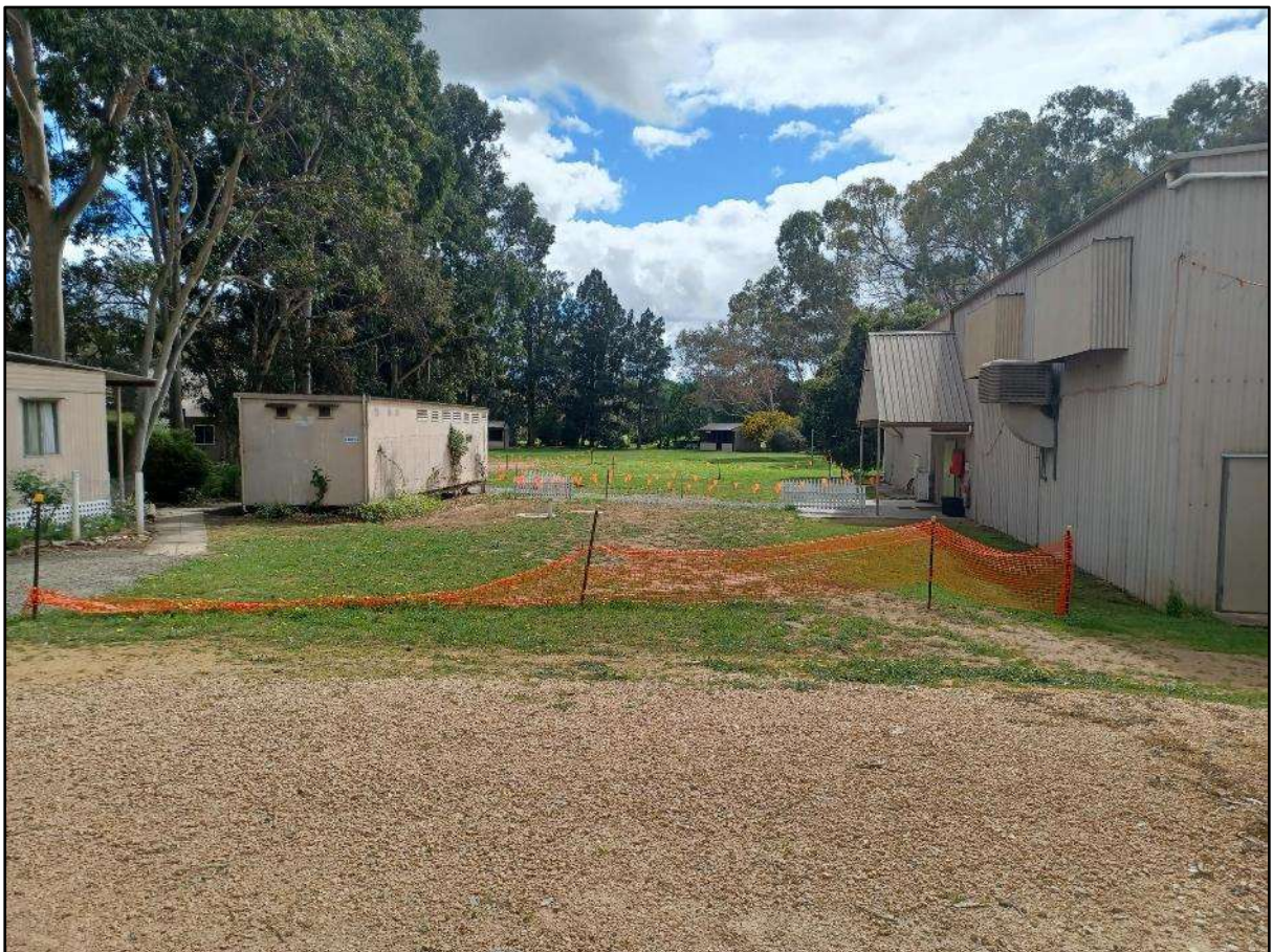
Figure 14: Site Photo – site of installation of new waste water system (approved by SA Health)
