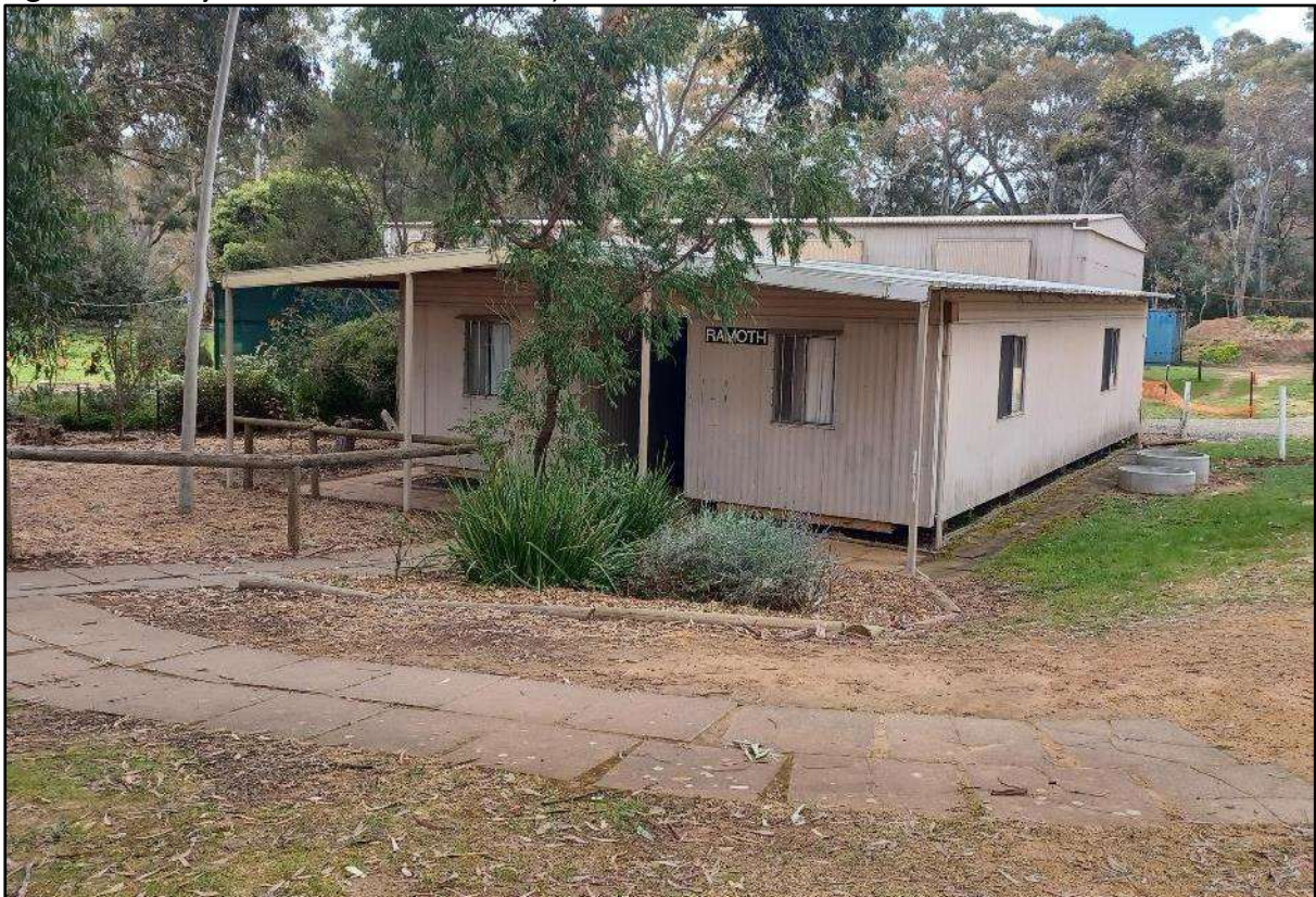
Figure 4: Site Photo – Dormitory H, to be temporarily relocated while replacement building is built
