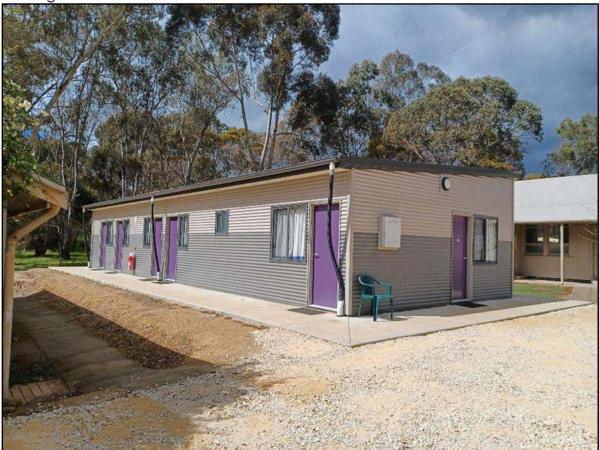
Figure 6: Site Photo – Dormitory C, already replaced
