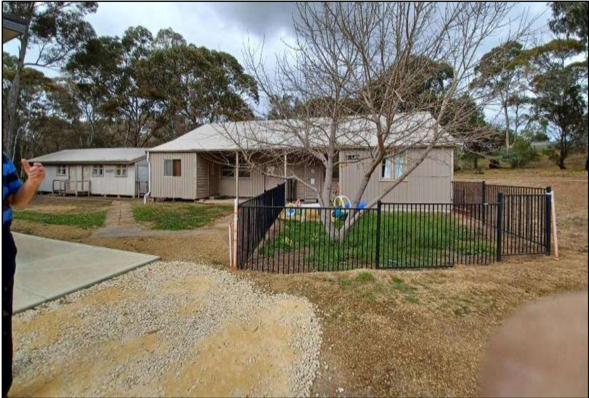
Figure 9: Site Photo – Former Classroom B, approved to be changed to dormitory as a part of 960/592/2018. This building is subject to current amendment to change internal layout
