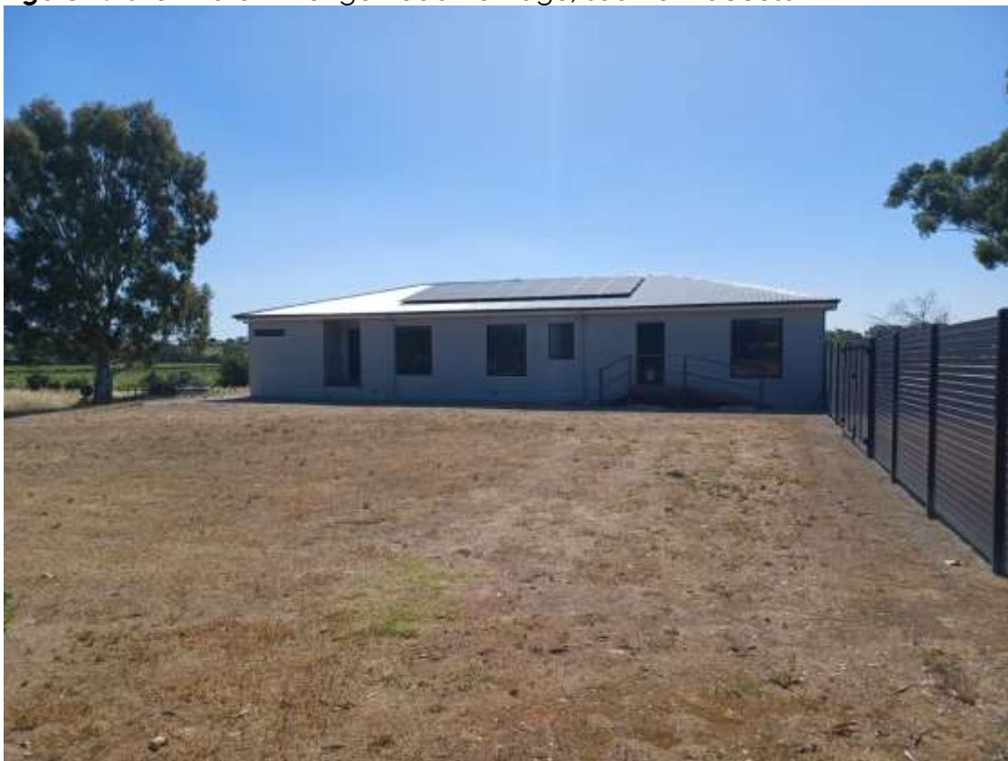
Figure 5: Site Photo of existing dwelling – Building façade
