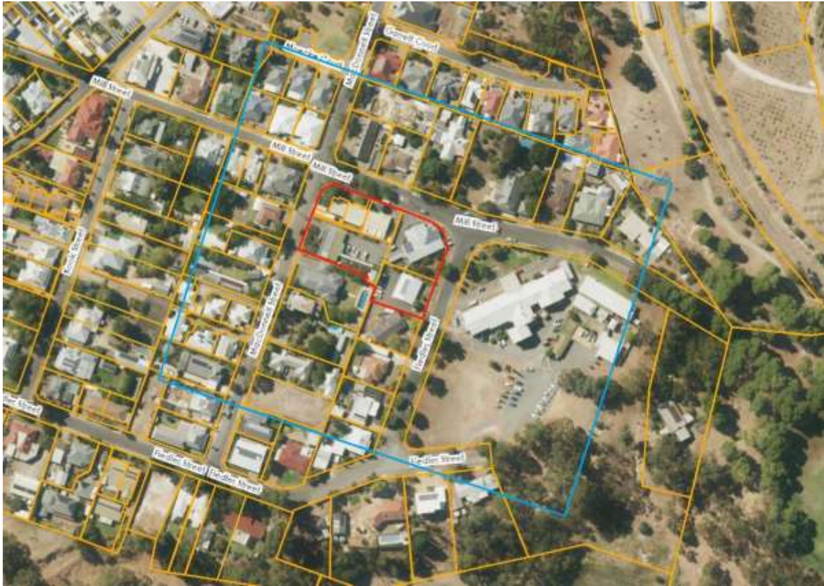
Figure 2: Aerial – Locality – subject site in red, locality in blue
