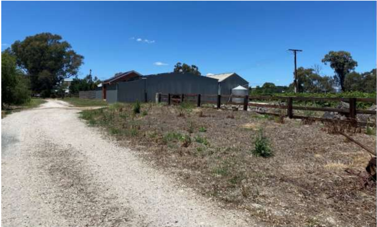
Figure 5: Site Photo – standing on opposite side of Old Mill Road Reserve, looking east towards winery and wine storage sheds
