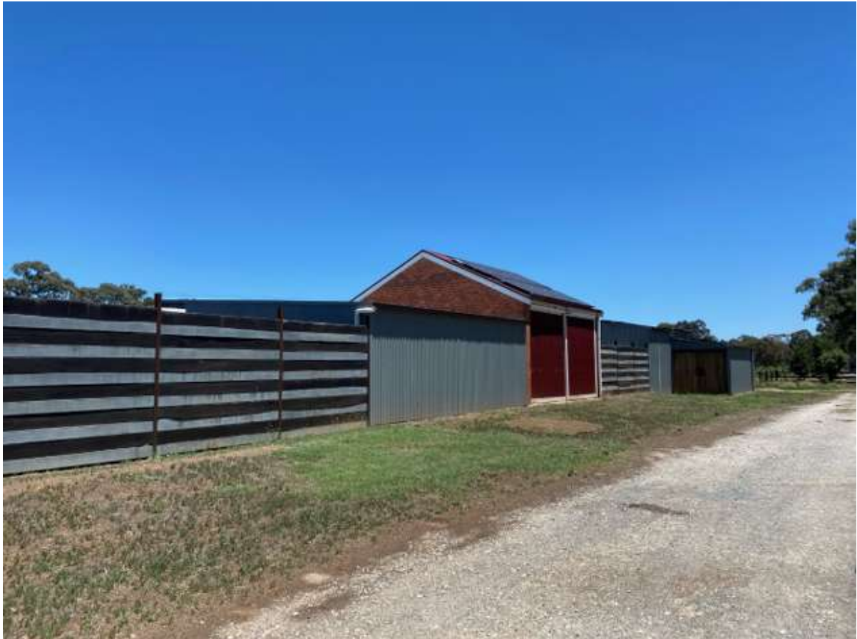
Figure 9: Site Photo - standing on Old Mill Road Reserve looking south-west, agricultural building will be located on the other side of the fence
