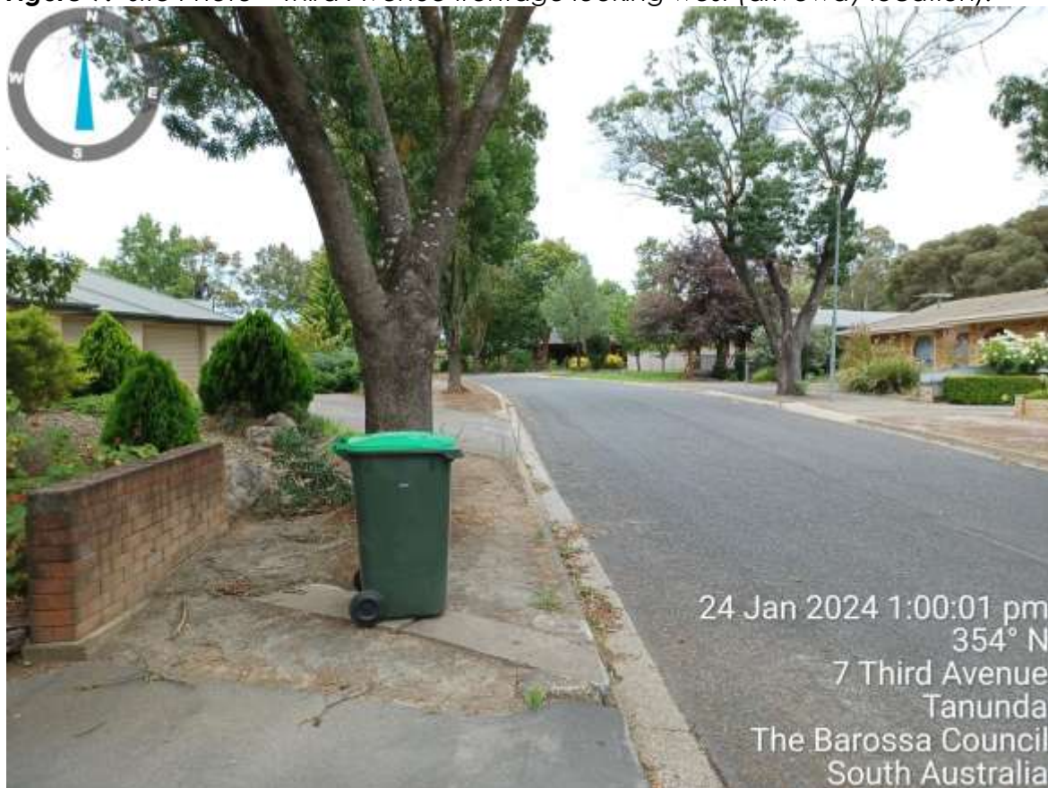
Figure 8: Site Photo – Third Avenue frontage looking north.
