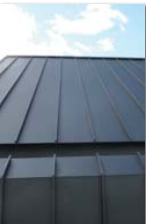
Roof & Walls Trimdeck Colorbond: Monument Planning Consent Refused The Barossa Council Application Number: 22027507
