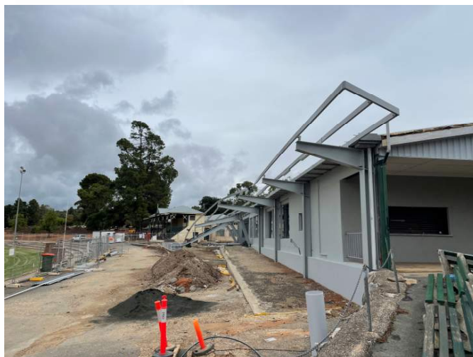
Photograph 1: The structural steel framed cantilevered canopy is located on the Eastern Side of the existing changerooms.
