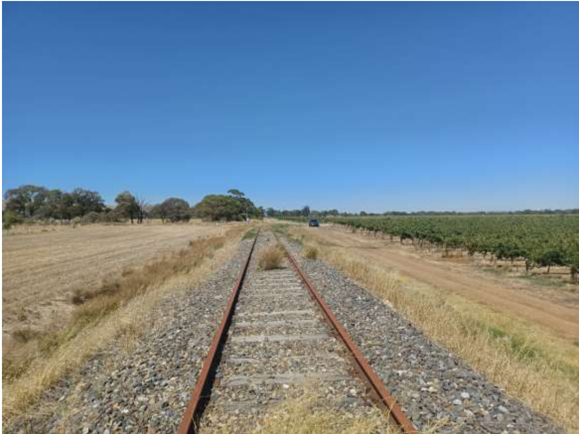
Figure 6: Site Photo looking south along railway corridor toward Rifle Range Road
