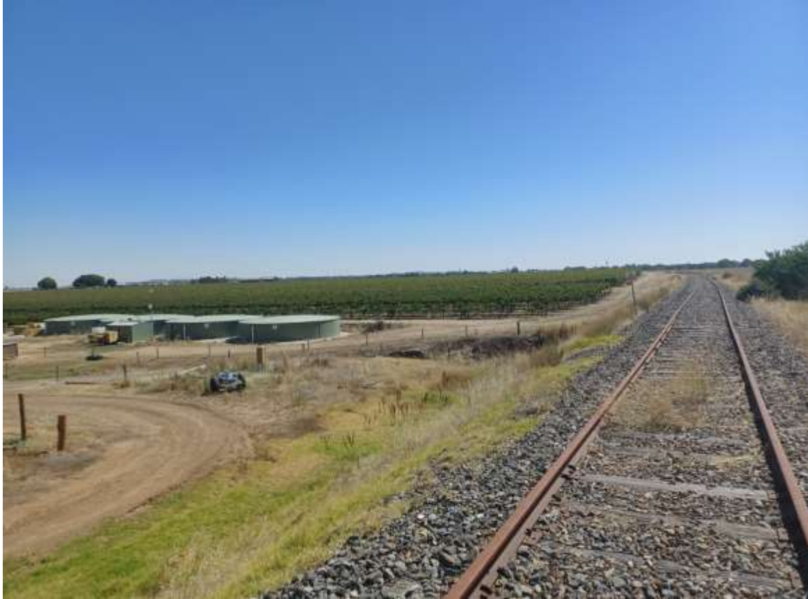
Figure 8: Site Photo looking north from railway corridor toward existing tanks
