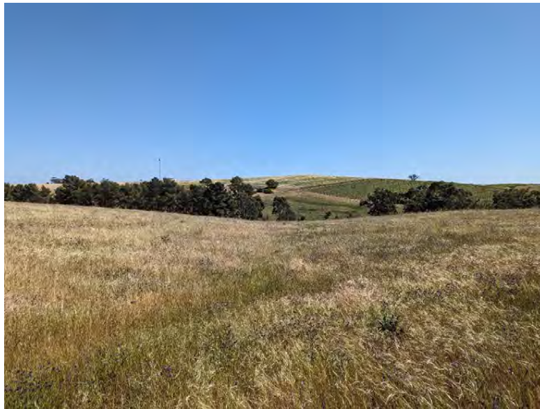
Figure A- 1: Northern wall of Old Salem dam
