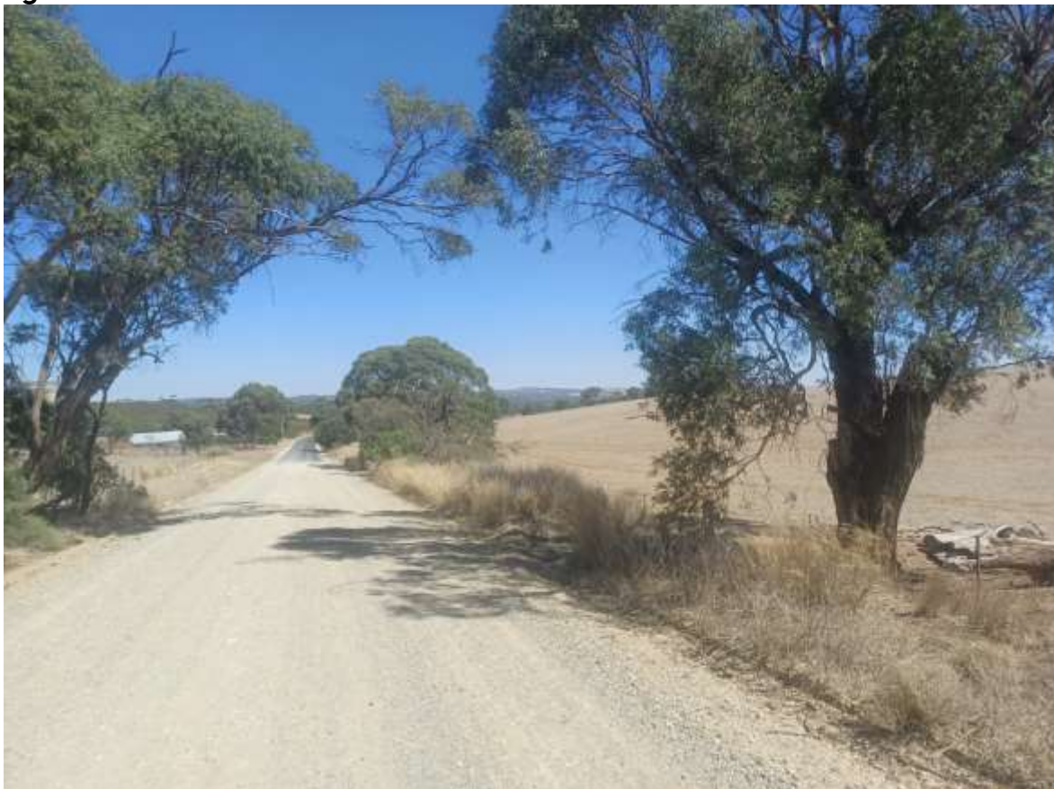
Figure 4: Site Photo – looking west along Duck Ponds Road adjacent site
