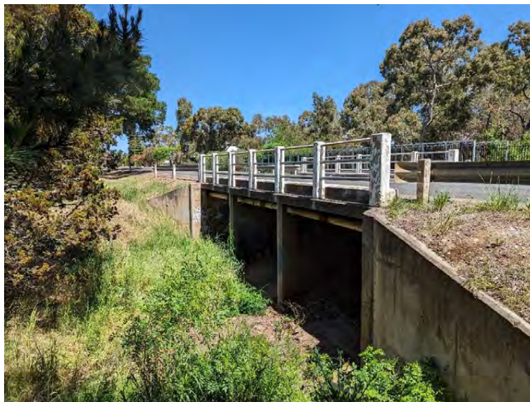
Figure A- 6: Stormwater culvert under Stockwell Rd.
