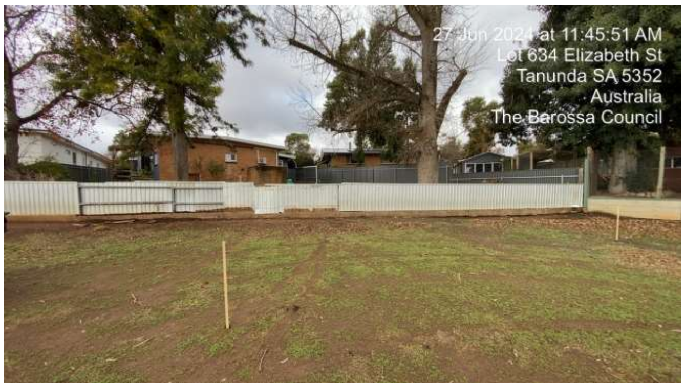
Figure 7: Site photo – Proposed building site facing east
