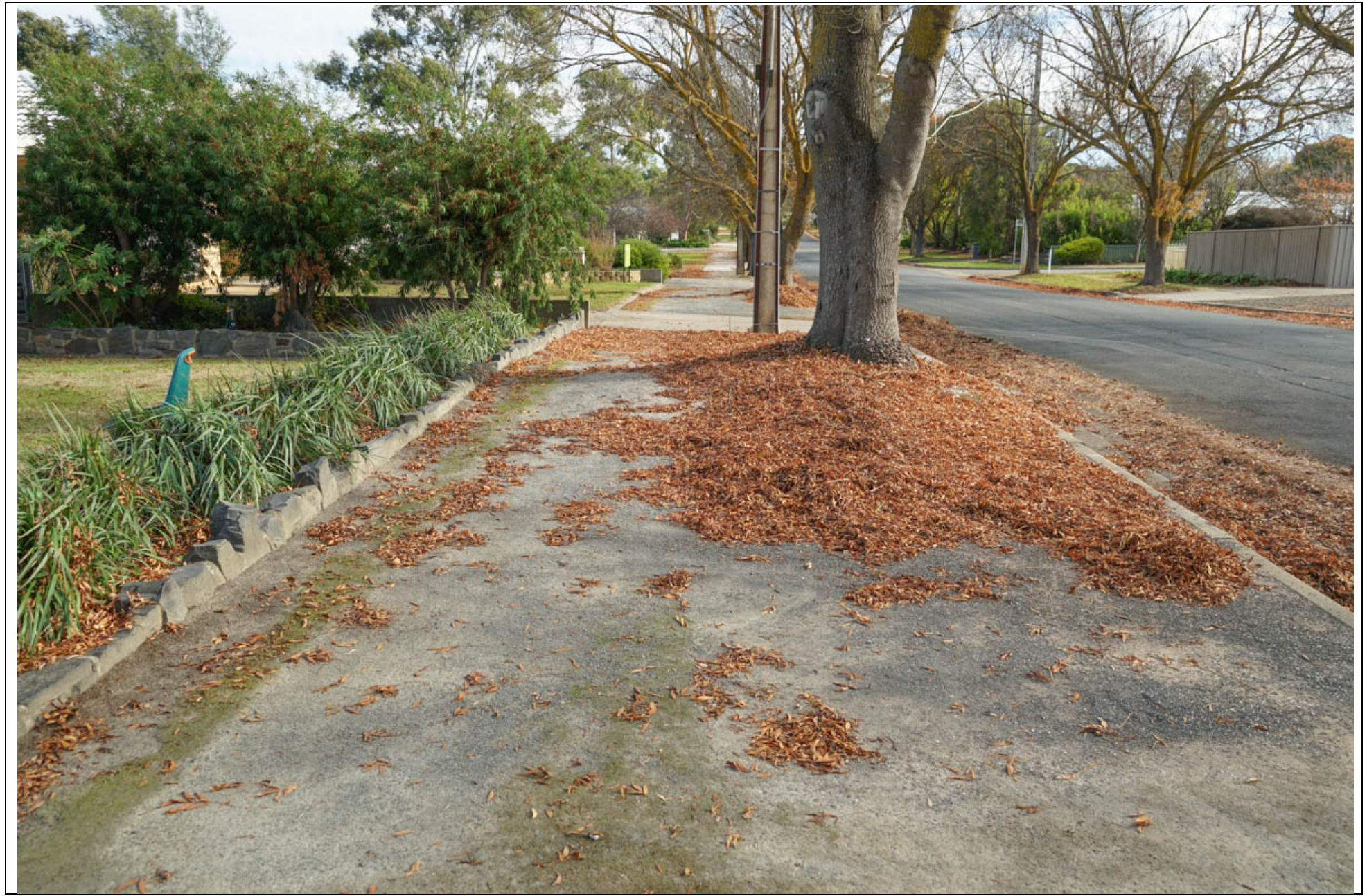
Photograph showing the dolomite verge area that is relatively level in form. Photograph also shows the small retaining wall located on the property boundary.
