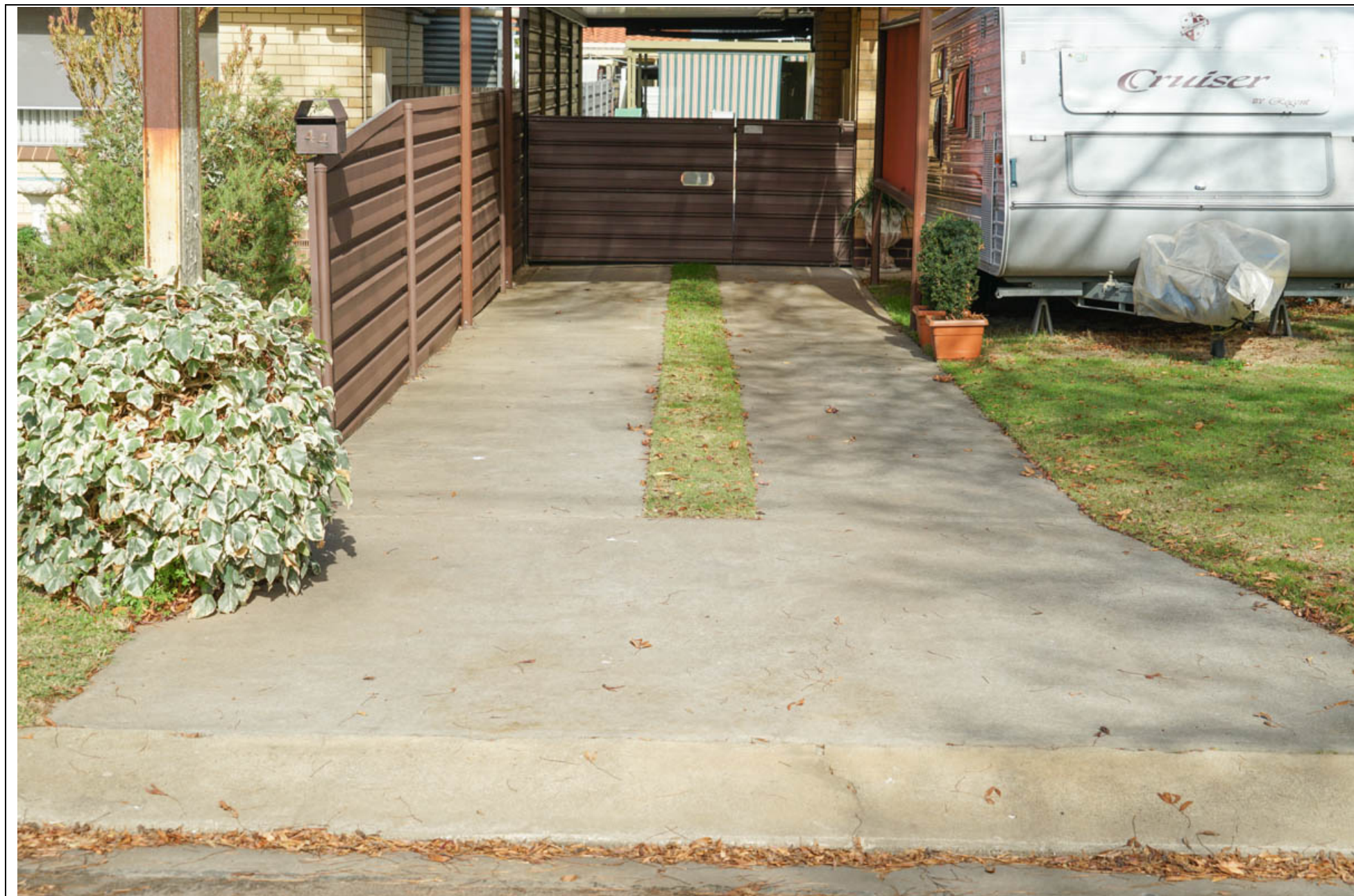
Photograph showing the cross over and driveway to the north of the tree showing no form of damage that could be related to tree root action.
