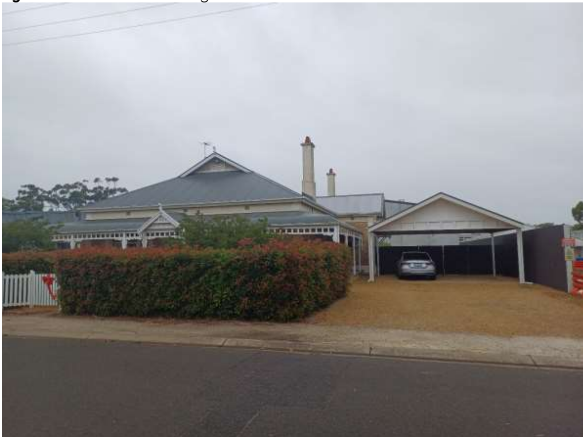
Figure 15: Site Photo – Looking south towards 4-6 Staehr Street
