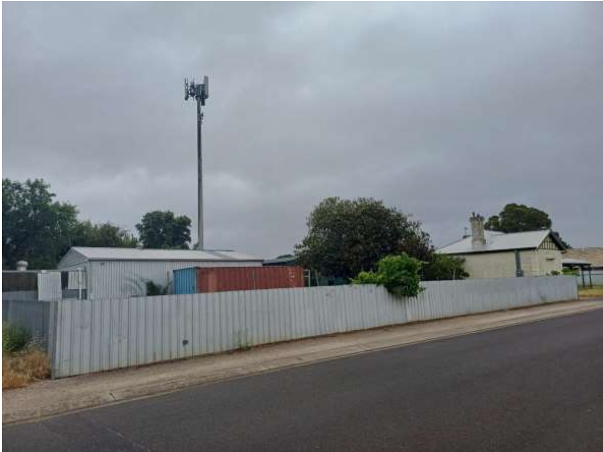
Figure 12: Site Photo – Looking north-east towards adjacent 5 Staehr Street
