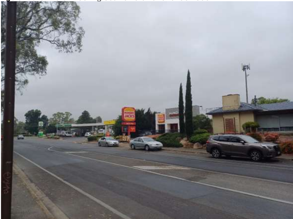
Figure 5: Site Photo – Looking north-east towards the Hungry Jacks
