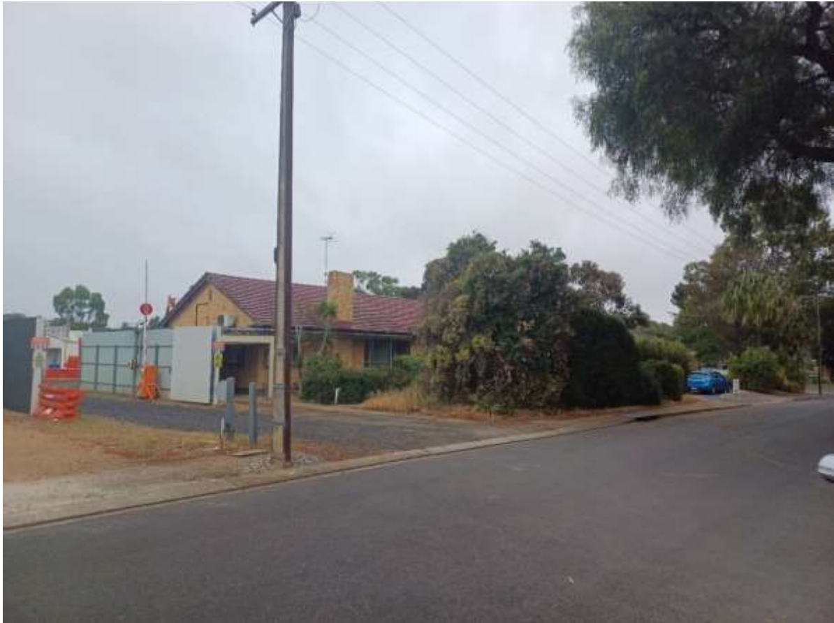
Figure 14: Site Photo – Looking south-west towards 2 Staehr Street
