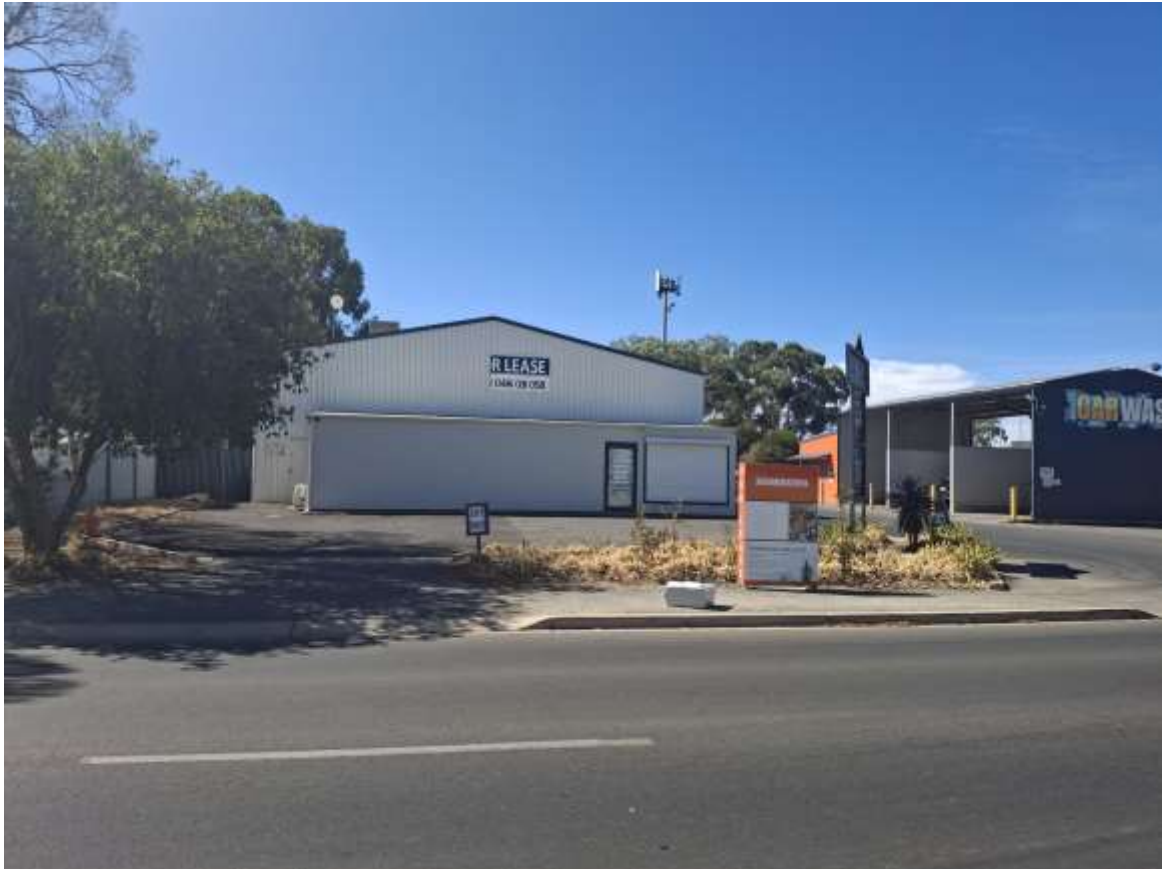
Figure 4: Looking north-east towards subject site from Para Road
