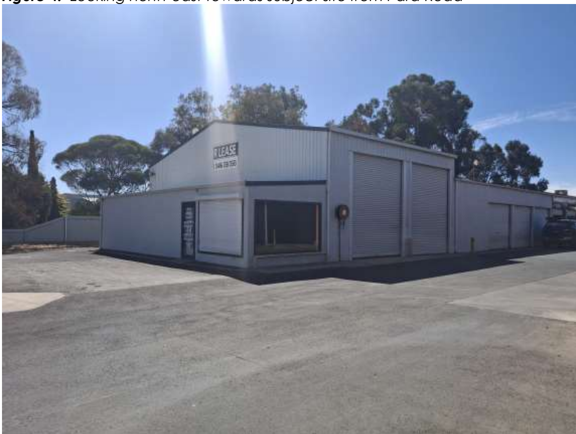
Figure 5: Looking north-east towards subject site from Para Road
