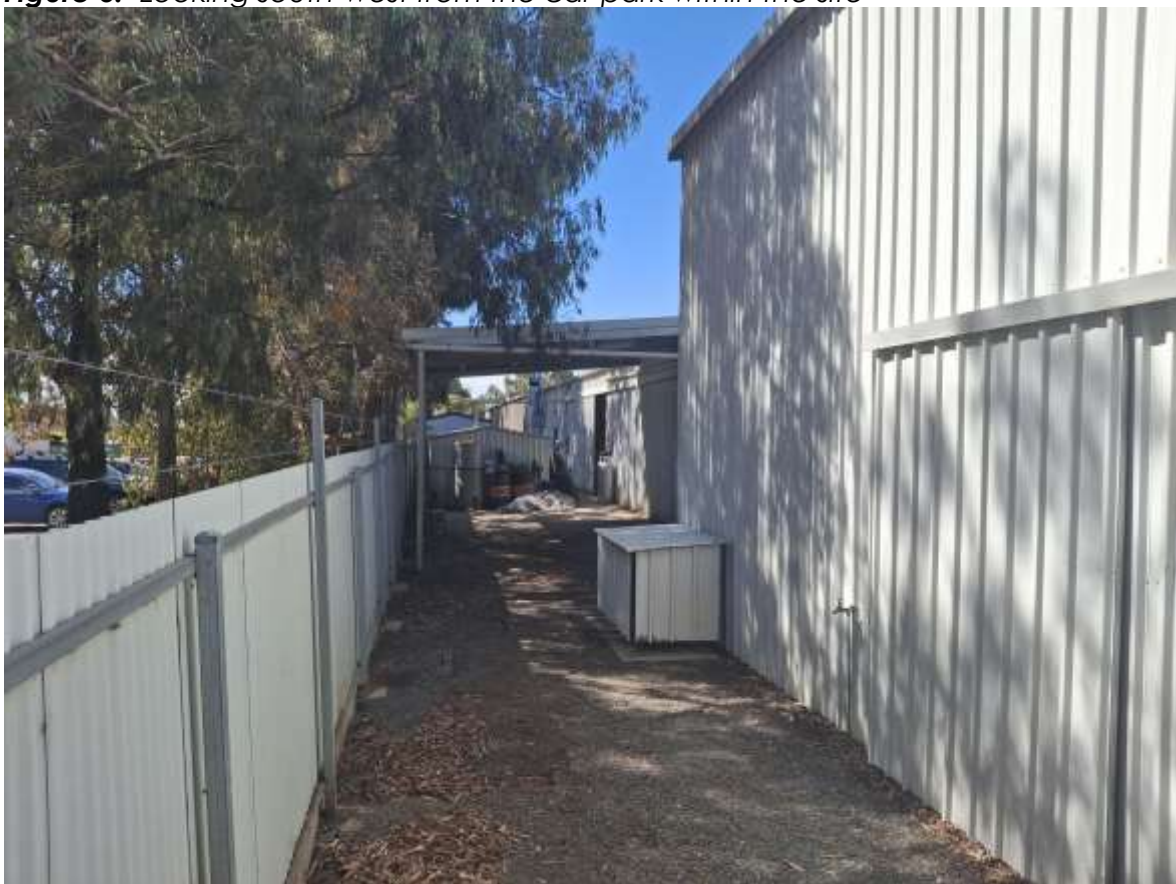
Figure 7: Looking north along rear of tenancy (western boundary fence)
