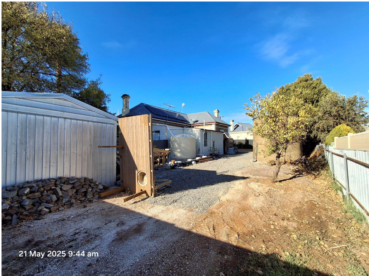
Figure 15: Site Photo – North-west corner of property looking toward rear of dwelling
