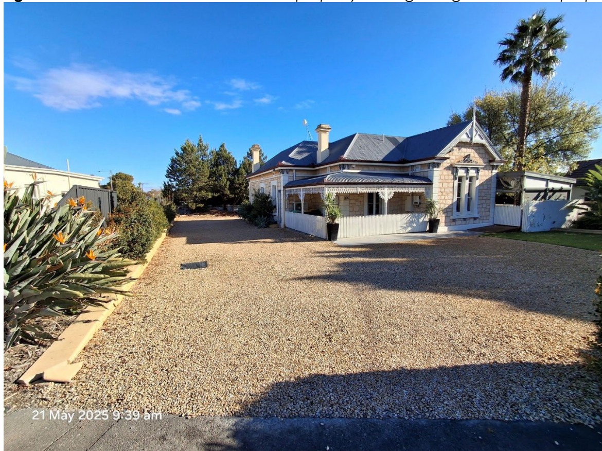
Figure 8: Site Photo – Front of property looking down driveway
