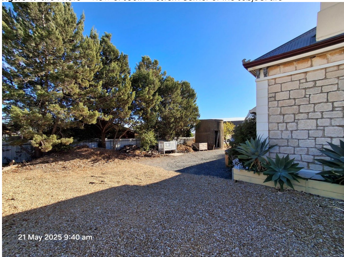
Figure 10: Site Photo – View of rear yard subject to dwelling addition
