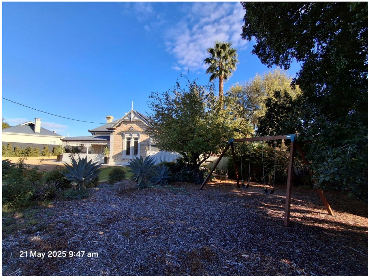
Figure 7: Site Photo – View from front of property looking along north side of property
