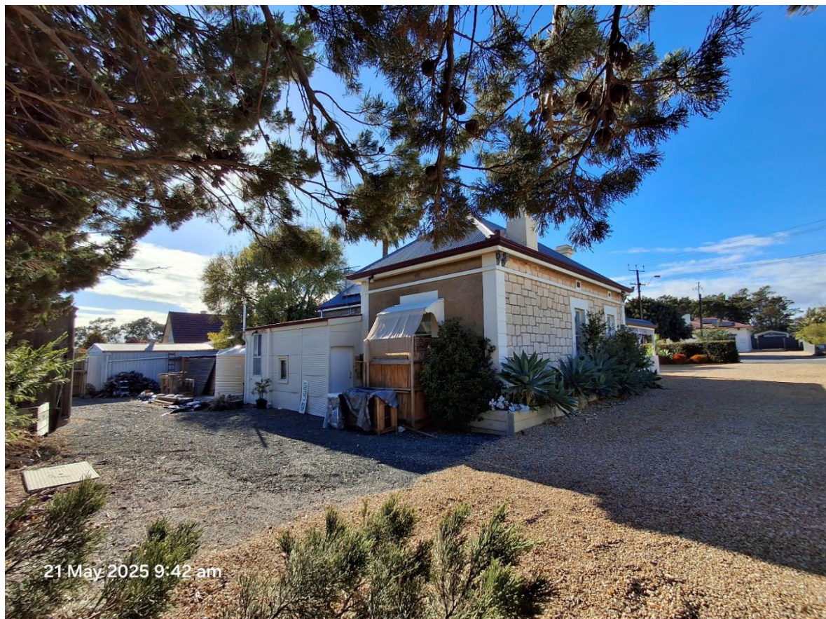
Figure 11: Site Photo – South-west corner of property looking toward rear of dwelling
