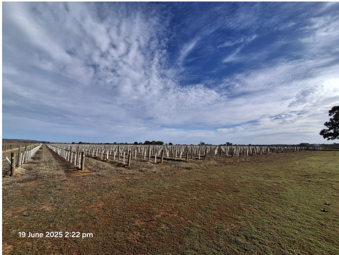
Figure 4: View from Penrice Road looking south-west towards frost fan 2
