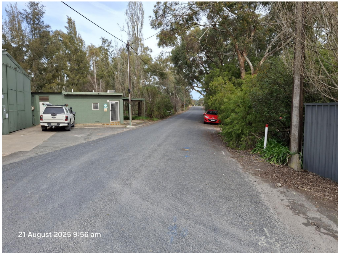
Figure 14: Site Photo – Rear of property carpark access looking south-west along William Street
