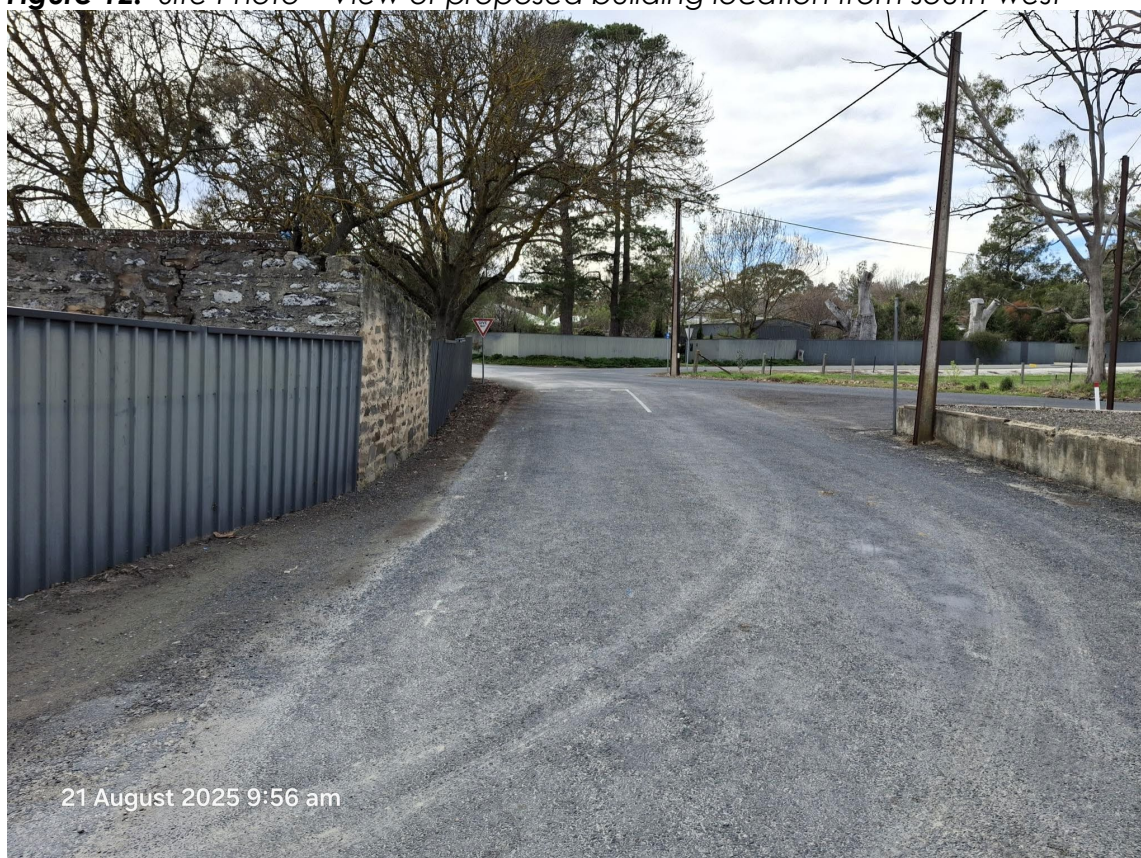
Figure 13: Site Photo – Rear of property carpark access looking north-east along William Street
