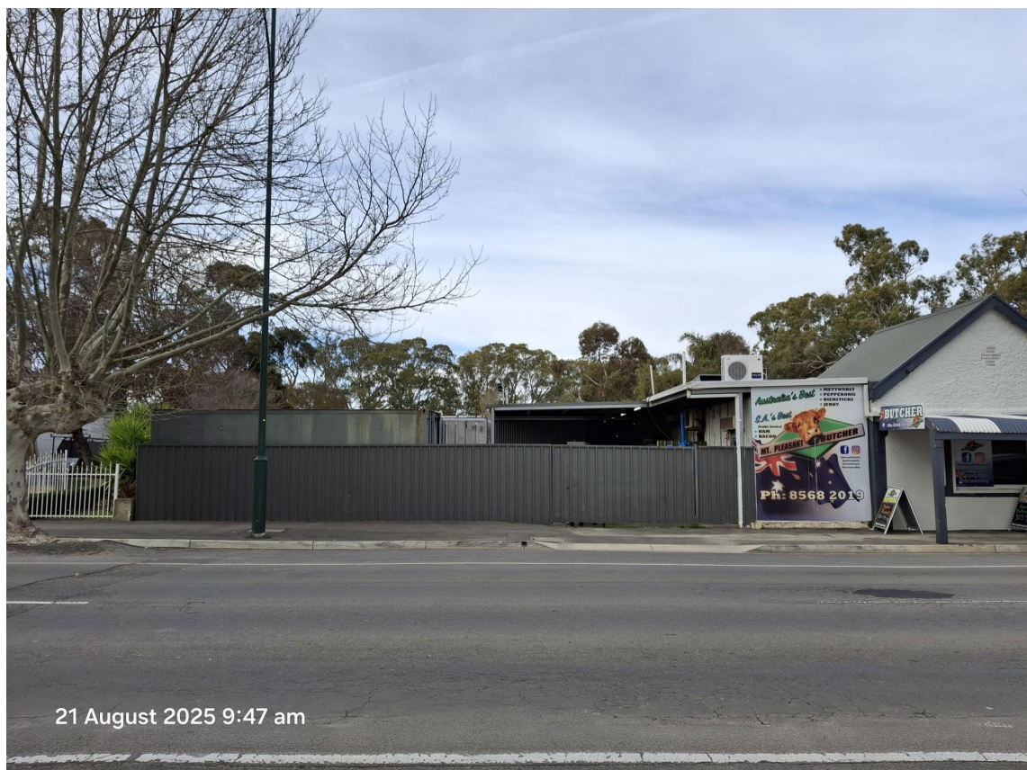
Figure 5: Site Photo – Looking south-east towards subject site from Melrose Street
