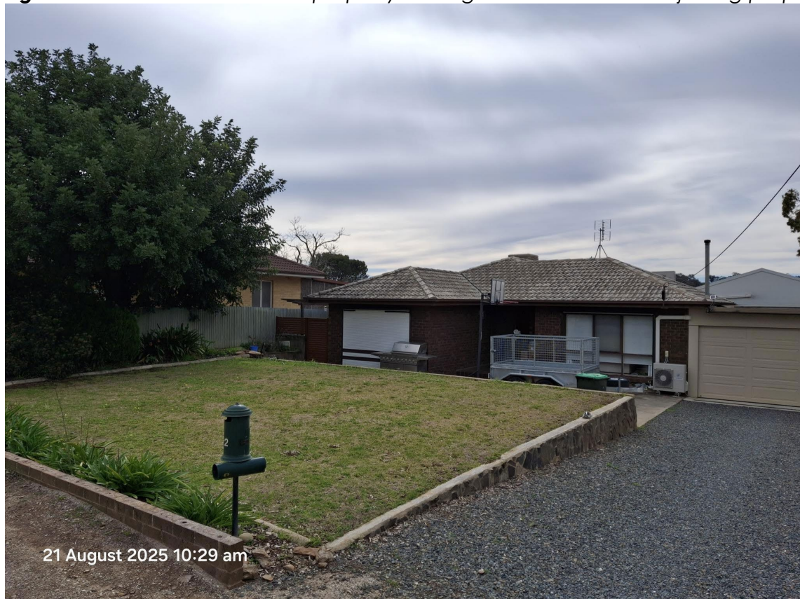
Figure 11: Site Photo – Front of property looking toward northern adjoining property
