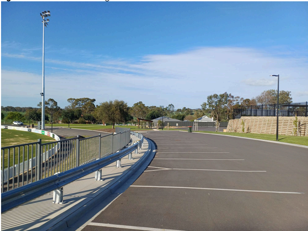
Figure 5: Site Photo- Looking east from car park
