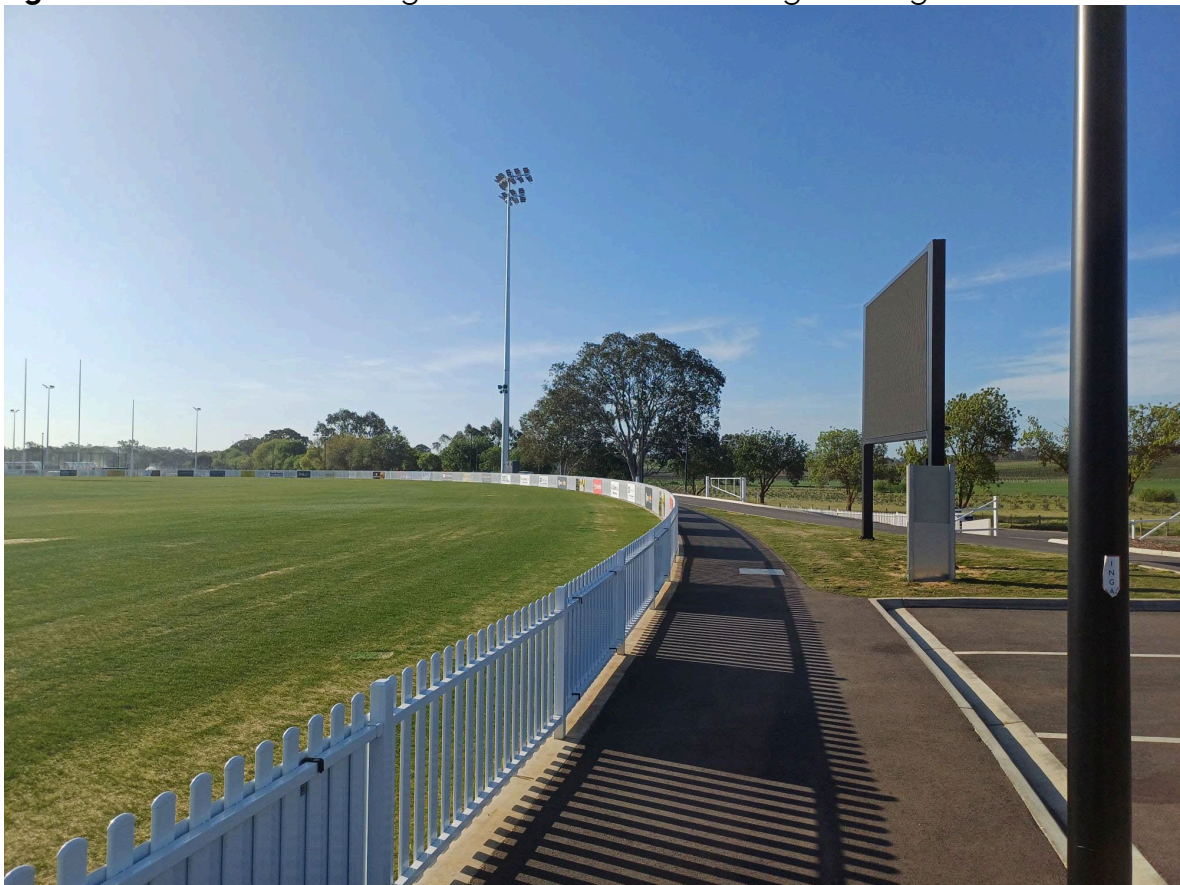
Figure 7: Site Photo – Looking north-east
