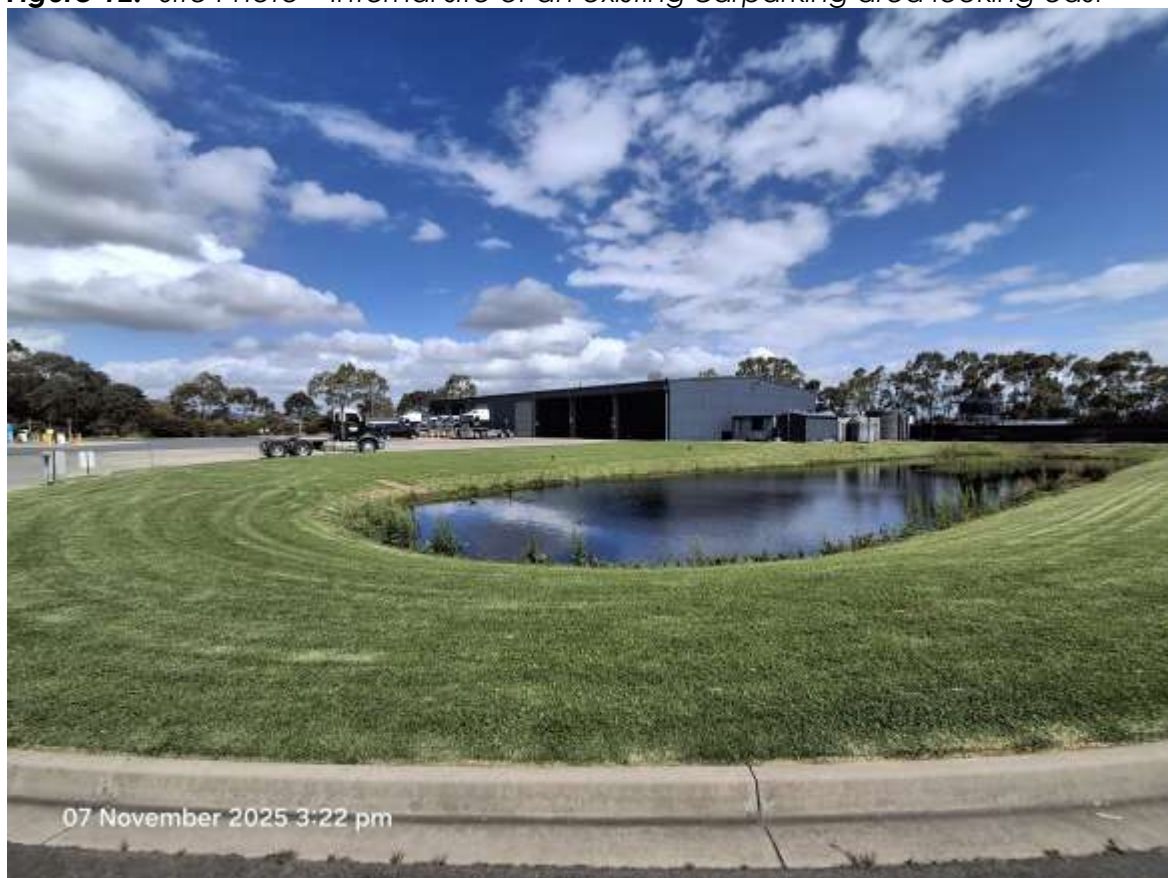
Figure 13: Site Photo – Internal site looking south over stormwater basin towards existing buildings
