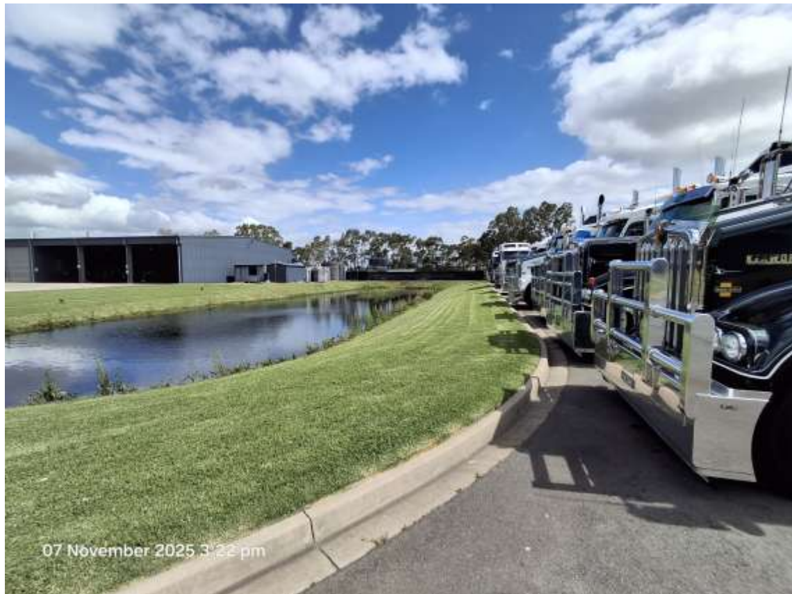
Figure 14: Site Photo - Internal site looking south over stormwater basin towards existing buildings
