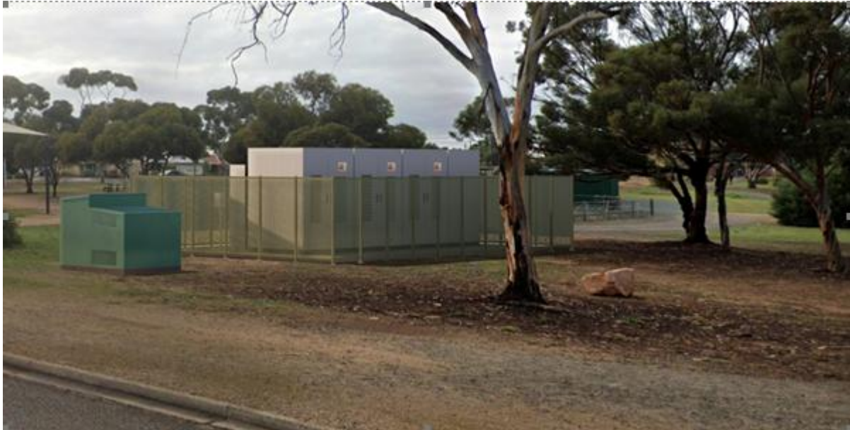
Figure 3 - ARTIST IMPRESSION ONLY of Battery unit in situ (Not Barossa location). The battery itself having dimensions of 7.5m long by 1.7m wide and 2.4m high, with total fenced area of 82.8m 2 .
