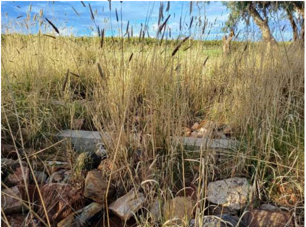
Figure 7: Site Photo looking south-west, further photo of the existing spill weir
