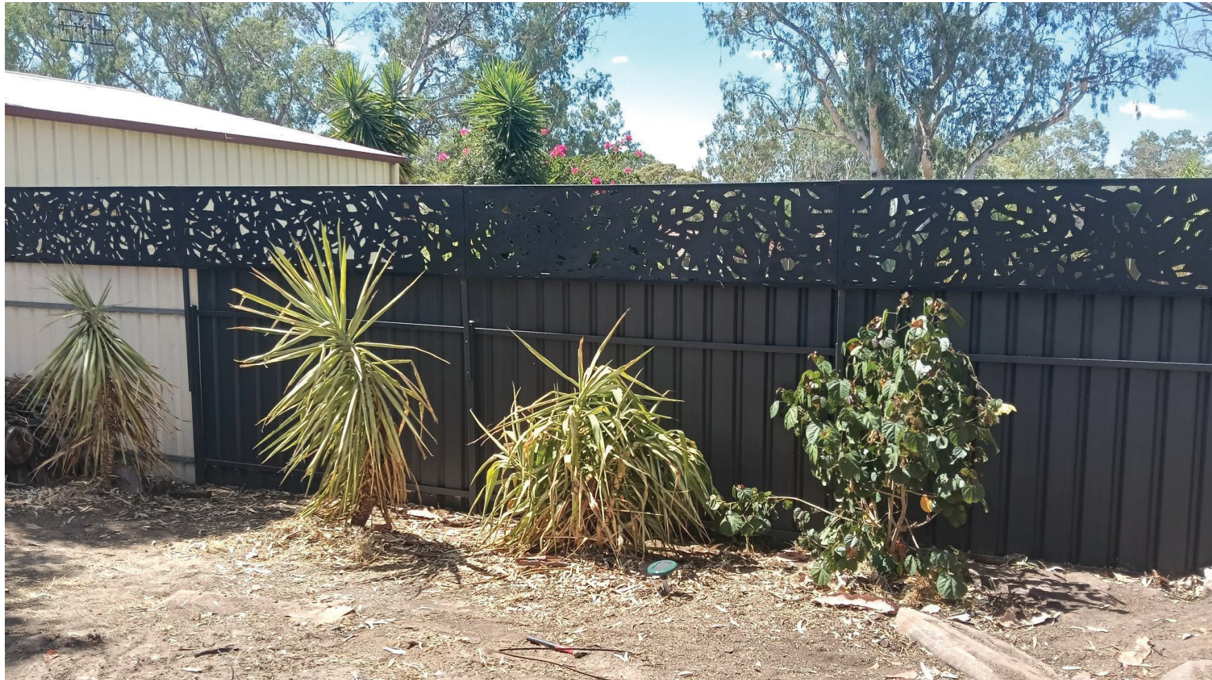
Facing southern boundary fence (fence extension installed to improve privacy and reduce overlooking)
