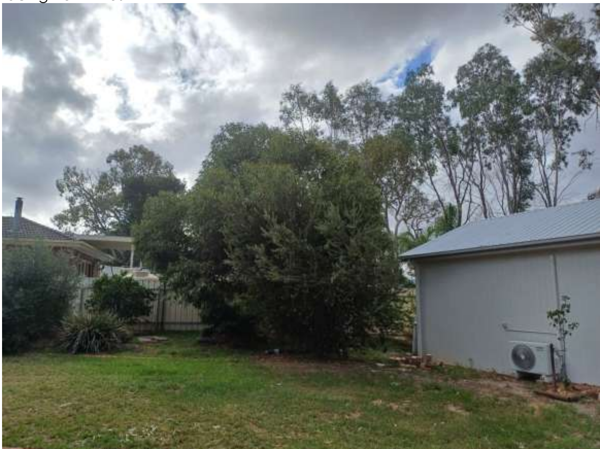
Figure 11: Site Photo – Shared tourist accommodation and ancillary accommodation facing north-west
