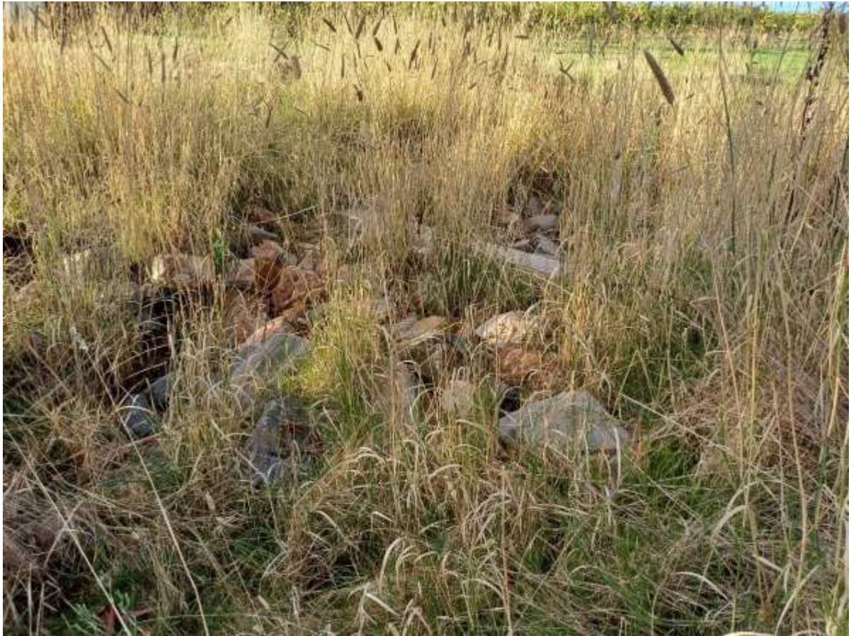
Figure 6: Site Photo looking south-west, toward existing spill weir and erosion stabilising rocks at the inlet to the existing dam
