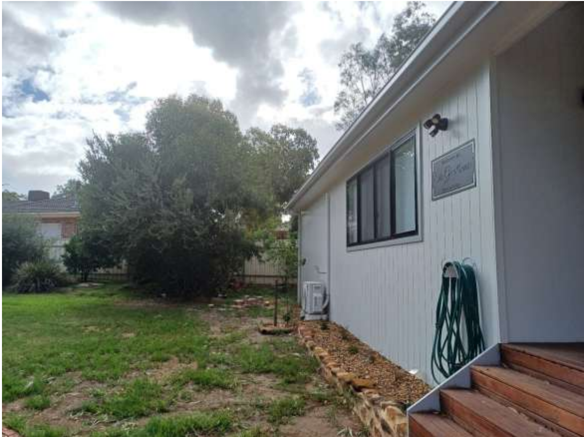
Figure 10: Site Photo – Shared tourist accommodation and ancillary accommodation facing north-west
