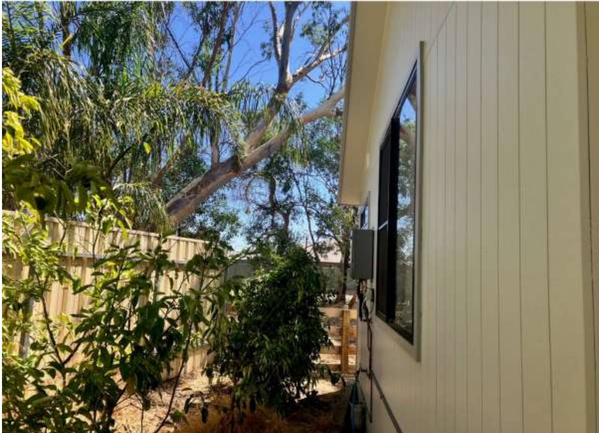
Figure 14: Site Photo – Bedroom window of the shared tourist accommodation and ancillary accommodation facing north-east
