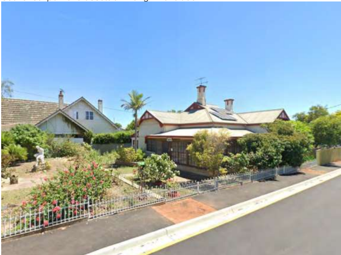
Figure 5: Site Photo – Looking south-west from Julius Street towards the existing single storey dwelling at 74 Murray Street, Tanunda
