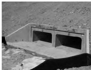
Small span box culvert with precast headwall
