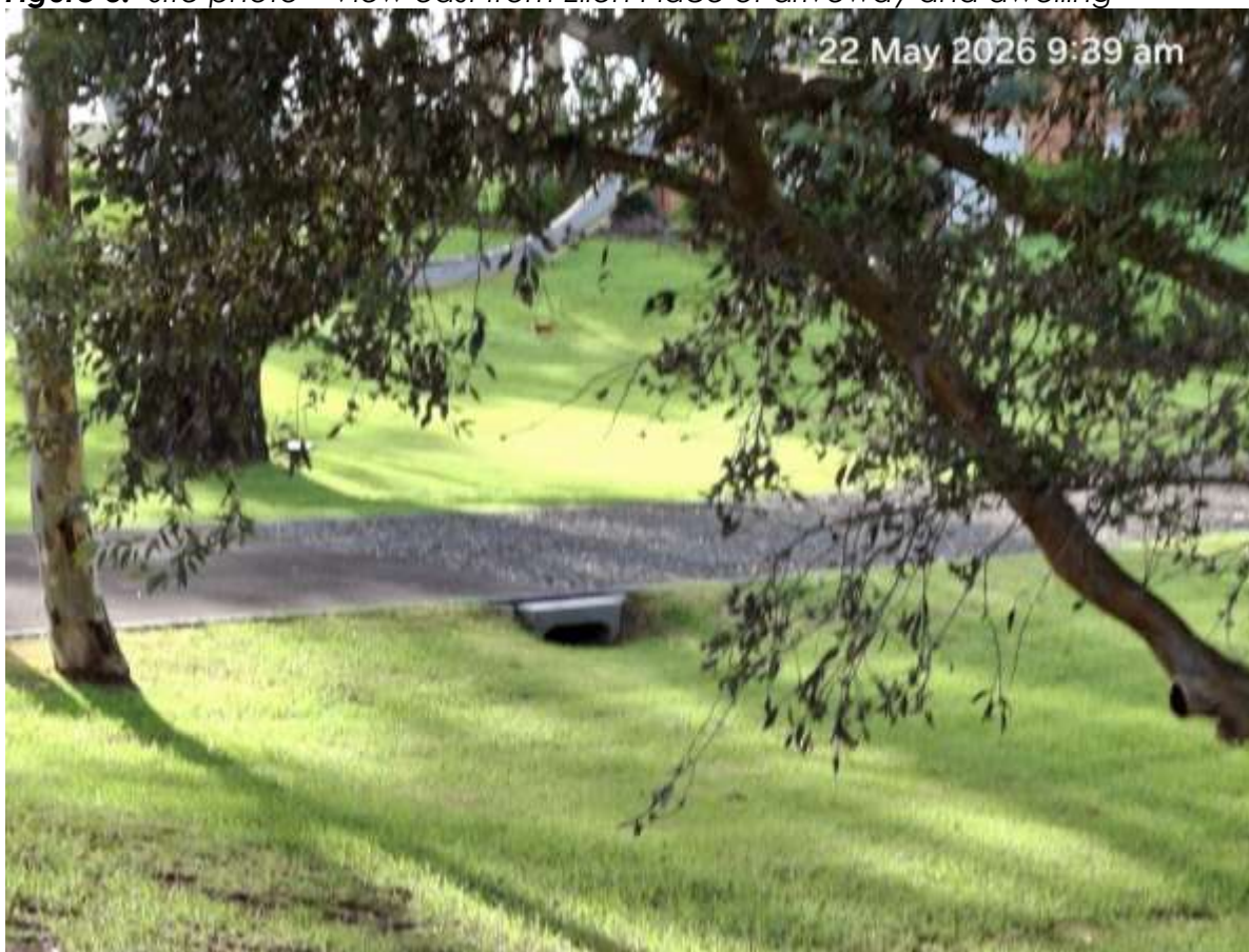
Figure 9: Site photo – Culvert of recently formed driveway access on Ellen Place
