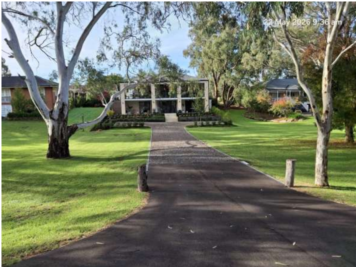
Figure 8: Site photo – View east from Ellen Place of driveway and dwelling
