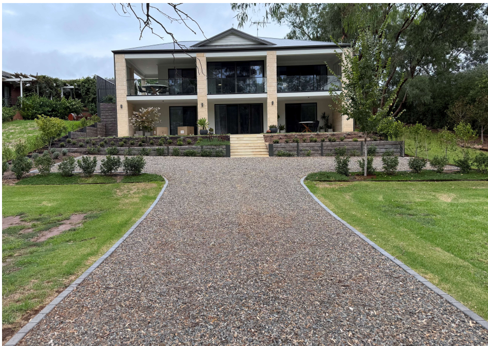
Image 3: Front Driveway as Constructed
