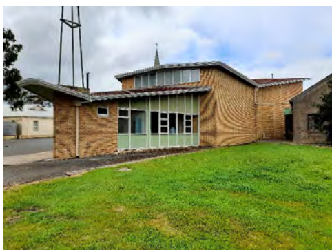
Southern and western elevations.
