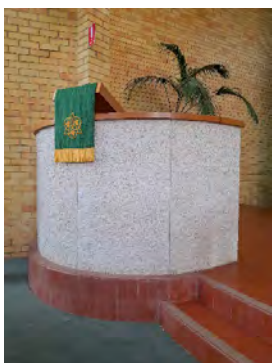
Pulpit in coarse aggregate concrete.
