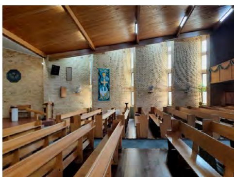
Nave showing sawtooth windows in side wall.
