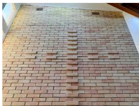
Cross motif in projecting stretchers on nave walls.
