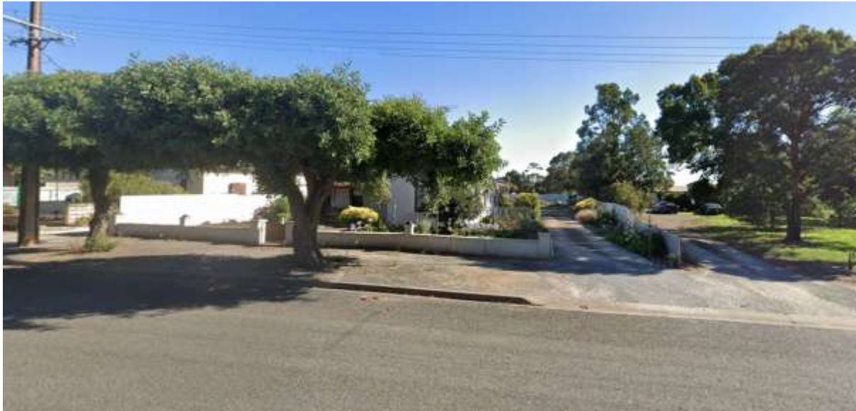
Figure 4: Site Photo – Road frontage looking at front of existing main dwelling
